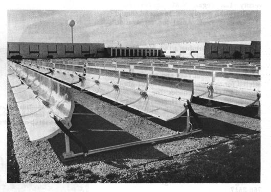
AT JOHNSON AND JOHNSON plant in Sherman, Tex. (above), solar collectors heat water to produce 100 psi steam. Steam passes around vats of liquid bleach used to bleach gauze. Campbell Soup Plant (below) uses rooftop collectors to produce 200°F water for washing cans.
